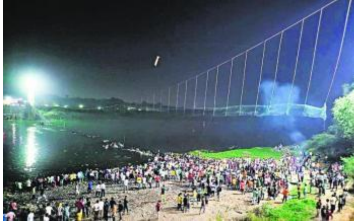
Morbi Suspension Bridge Collapse on 30th October 2022
